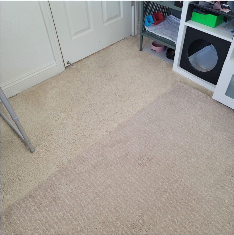
Indoor (room 1, upstairs)
